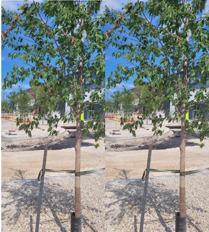
Example of conversion of grey infrastructure to green infrastructure – St. Vital Mall parking lot
